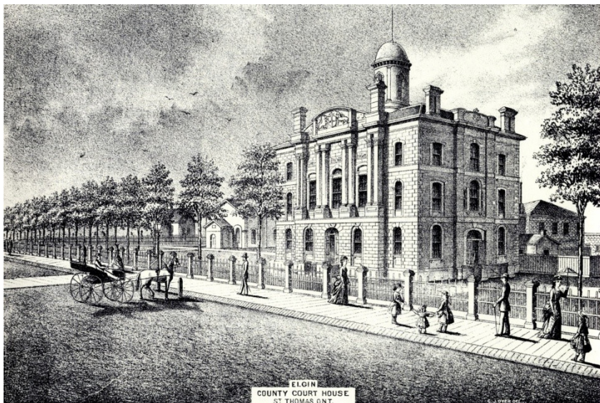
Figure 32- Elgin County Courthouse - 1877
